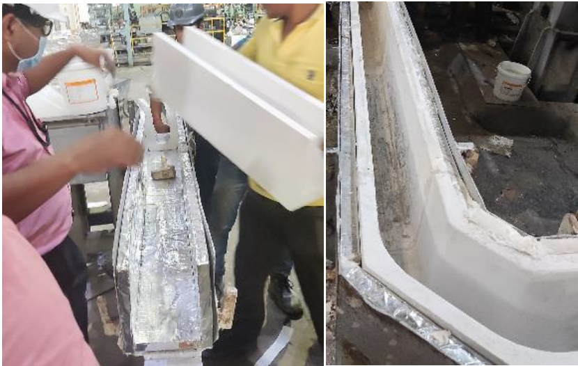
Figure 2 Installation of WDS Ultra Board
