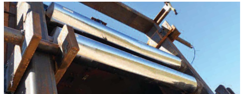
Pipe system after second explosion test.
